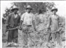
ABOVE: Black workers help build Muny; the photo is from the collection of Tinsley Penick, son of legendary golf instructor Harvey Penick.
